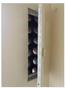
Figure 111: Anhalt (1-bedroom unit) – Interior view of bedroom window ventilation system
